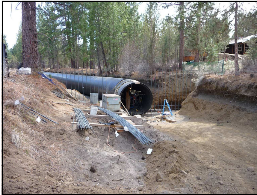
Tumalo Irrigation District is replacing over 6 miles of open canal sections with large diameter conduit. This latest phase of construction will save over 530 acre-feet of water once lost to seepage.
