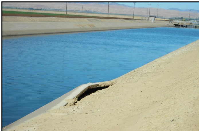
Land subsidence along the Delta-Mendota Canal, Western San Joaquin Valley (CALIFORNIA). Photo Credit: Michelle Sneed, USGS.
